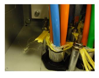
WRAP 1/2 OF THE DIELECTRIC STRENGTH MEMBERS TWICE AROUND EACH STUD AND BETWEEN THE TWO WASHERS. TIGHTEN WITH A NUT.
